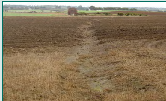
Plate 59 Spoon drain installed to direct surface water off a paddock, northern Tasmania. Source: Finnigan, J. (2008)
