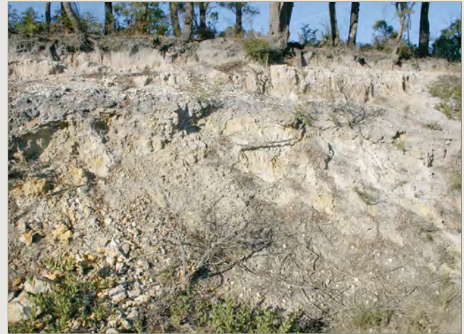
Plate 11 Deeply weathered layered/fractured sediments near Bridport. Source: Hocking, M. (2008)
