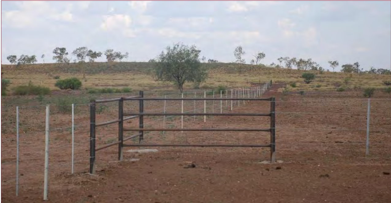
Figure 32: Two corner assemblies using pipe rail fencing, cemented into the ground
