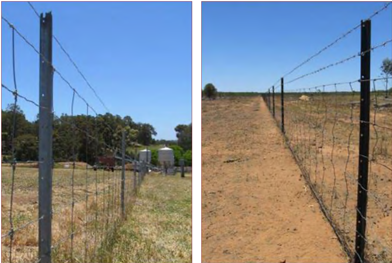
Figure 34: Examples of well-constructed ringlock fences
