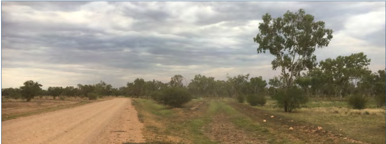
Figure 25: Example of well-constructed flat-bottom drain, Kimberley Region, WA
