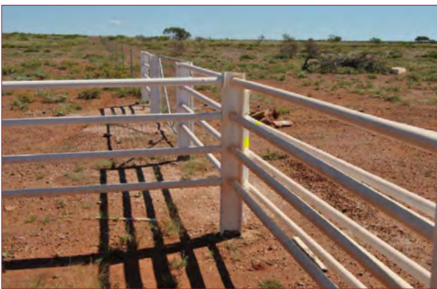
Figure 33: Fence strainers at a gate
