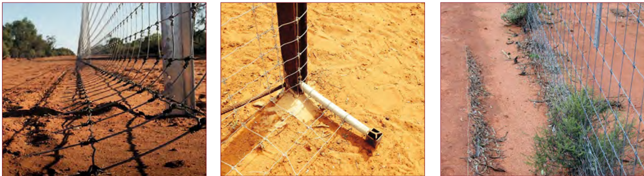
Figure 37: Examples of different types of aprons for exclusion fences
