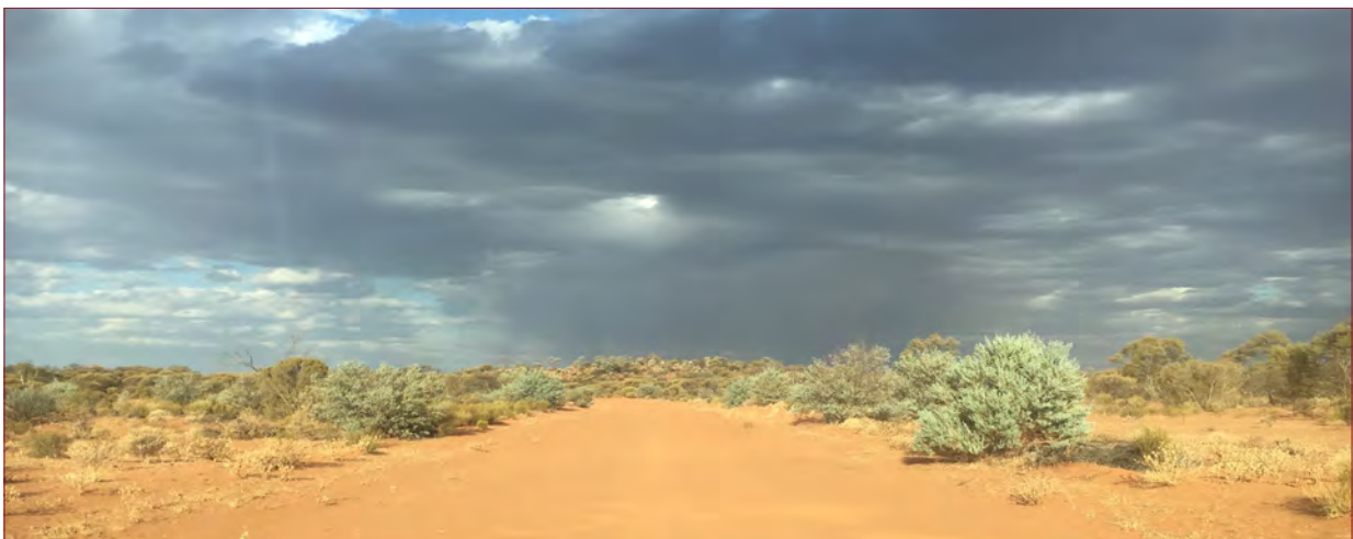
Figure 17: Example of a well-constructed road on flat surface, Murchison Region, WA
