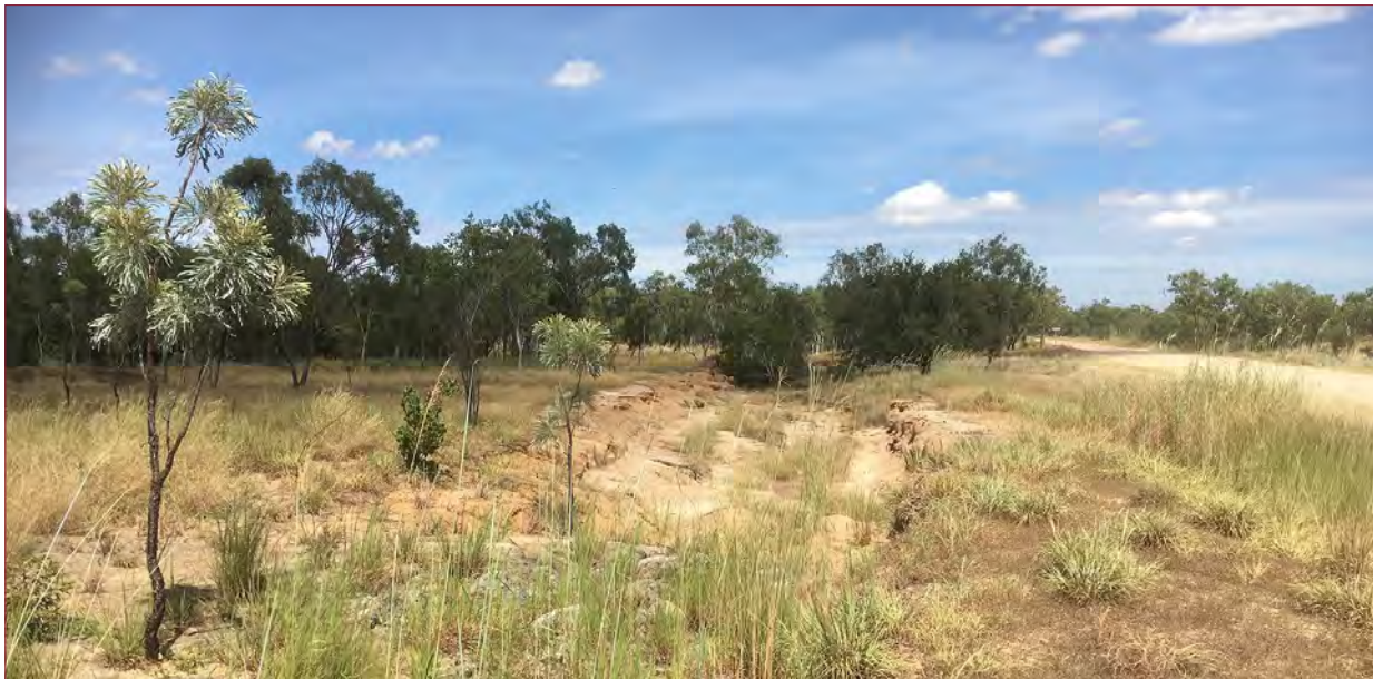
Figure 22: Erosion gully created by a windrow beside Gibb River Road, Kimberley Region, WA
