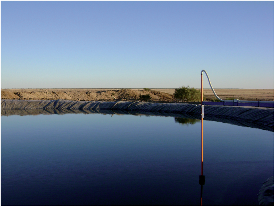
Figure 9: Example of dam liner used to control seepage losses
