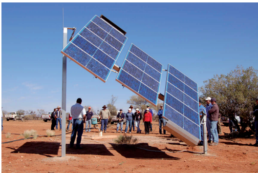
Figure 3: Solar pump used to push water up a hill
