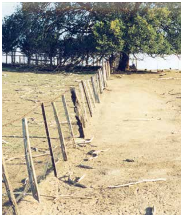
Existing fence lines can be used for one or more sides to minimise costs
