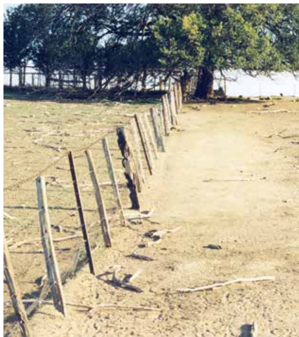
Existing fence lines can be used for one or more sides to minimise costs.
