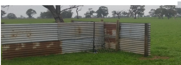
Figure 6. T-shaped corrugated iron shelter.
